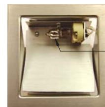
Relamp Step light fixture ONLY with OSRAM MINISTAR® 10W / G4 / 12V lamp with reflective coating in the up position.
